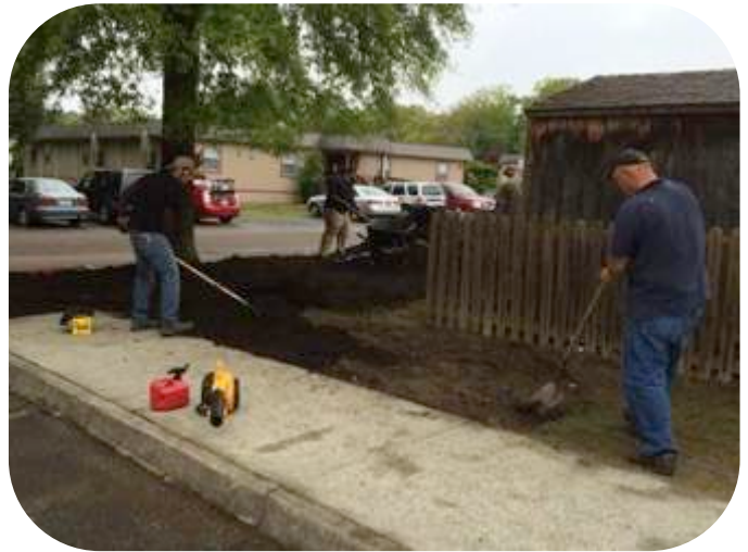
Clint and Dale hard at work spreading mulch and digging trenches
